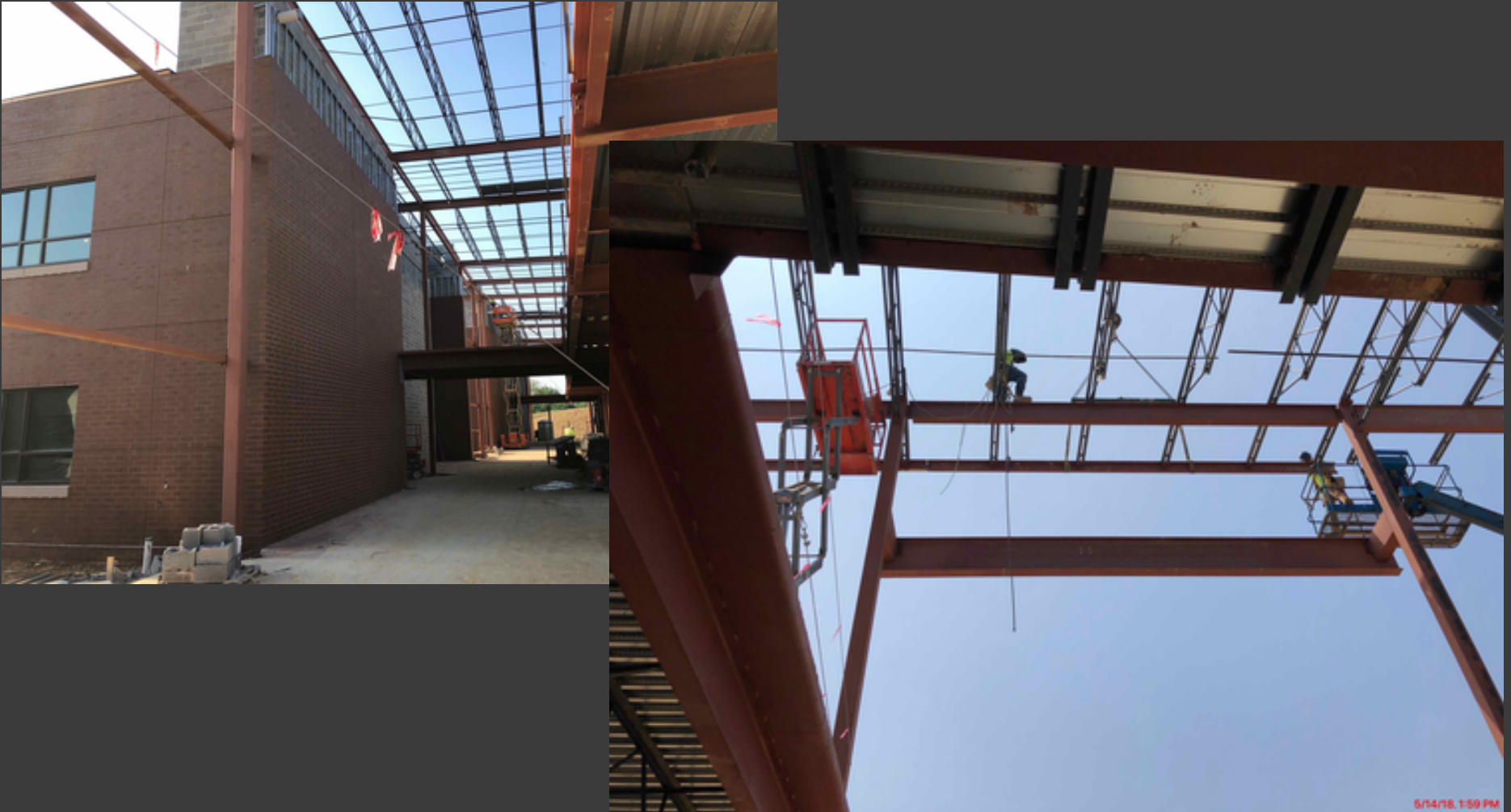
Steel Joists Installed in Main Street
